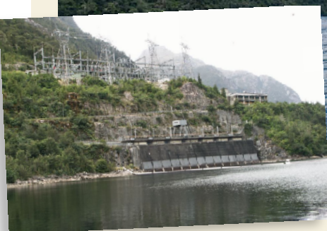
Manapouri Power Station - inlaat water.
