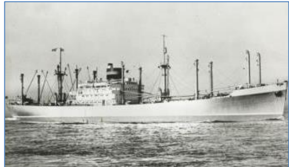
ss. Overijssel (C 3 -S-A 5 ) 8500 pk van Westinghouse Electric, 18 kn.
